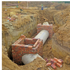
WE ALSO DO DEMOLITION, STORMWATER CONSTRUCTION, AND MAJOR SERVICES.
